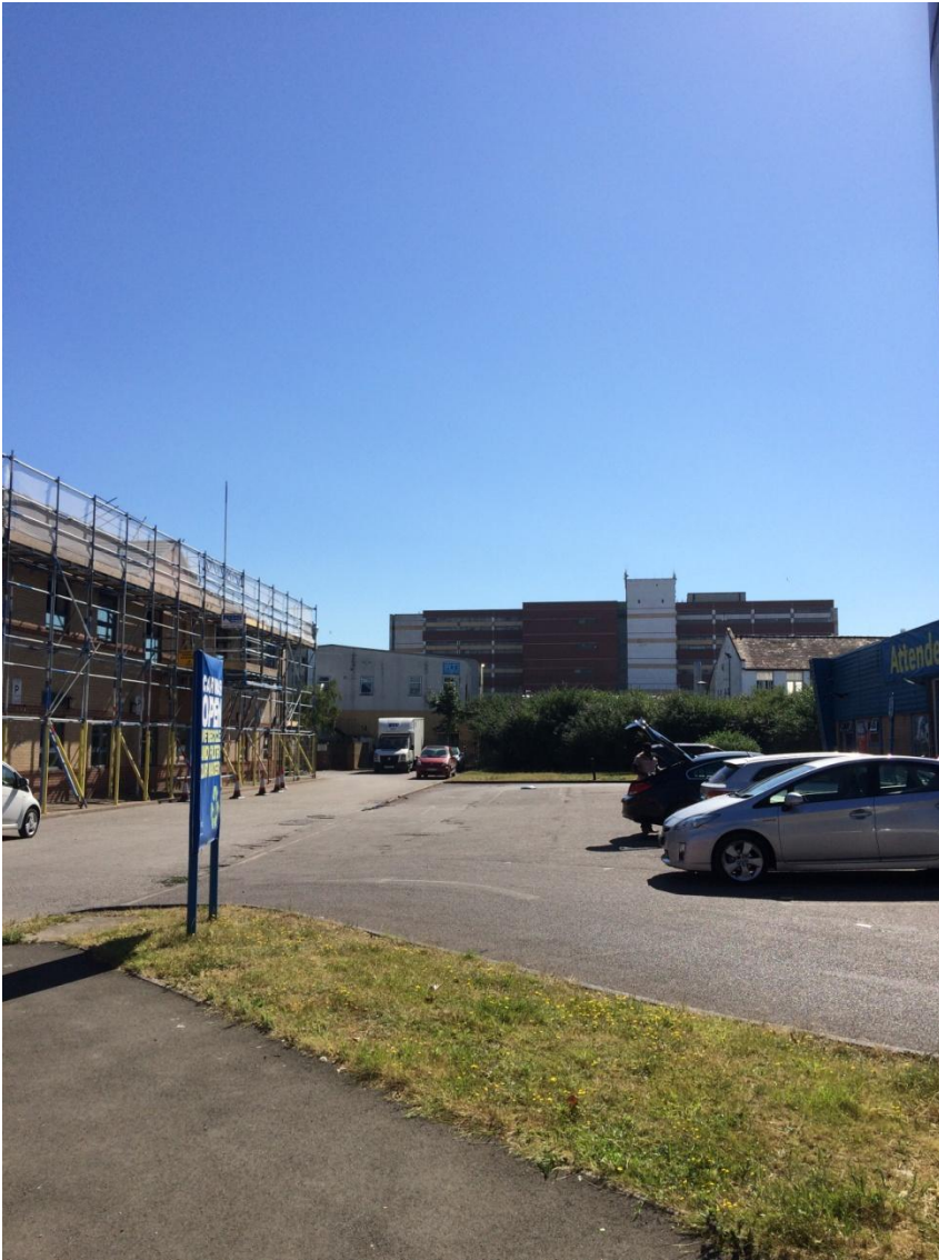
Existing car wash
