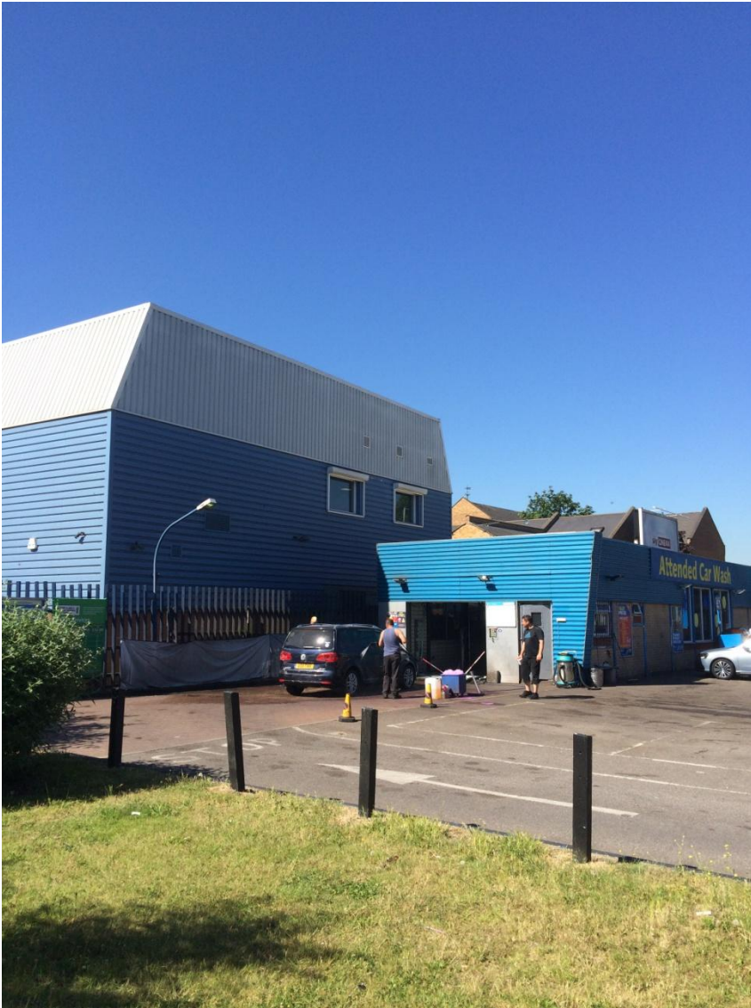
Existing car wash
