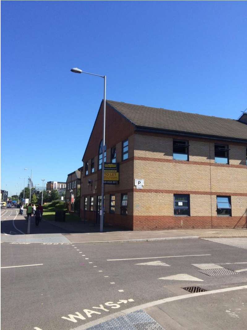
Adjacent office block
